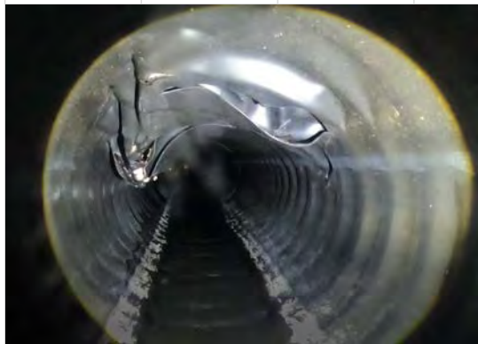
1) Damage between 20LF and 25LF from 3C.
